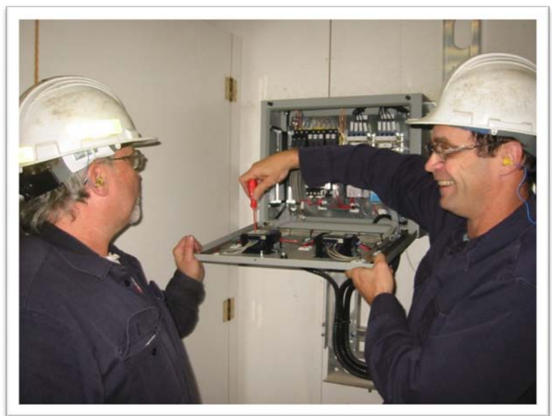
Installing new electrical meters. Photo courtesy of Flakeboard.
