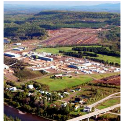
Twin Rivers Plaster Rock lumber mill. Photo courtesy of Twin Rivers. Plaster Rock produces dimension lumber and studs for residential and commercial construction applications. By-product softwood chips and biomass are used internally at its pulp and cogeneration operations in Edmundston, providing a secure source of SFI® certified wood fiber.
