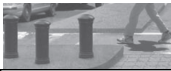
Bollard Protected Median
